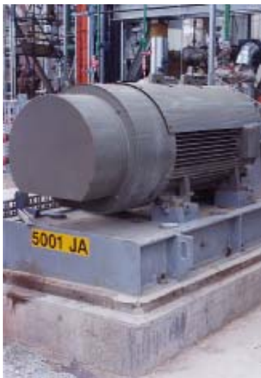
Grouting of motor baseplate with Conbextra EP products
